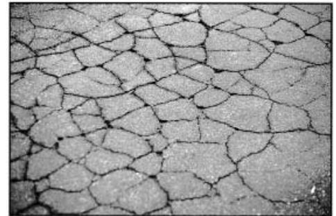
Figure 1: Chicken wire/alligator pattern cracking typical in fatigue cracking
