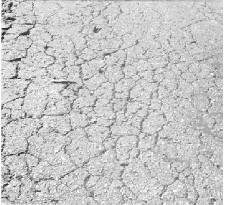
Figure 2. Alligator Cracks (photo courtesy The Asphalt Institute)
