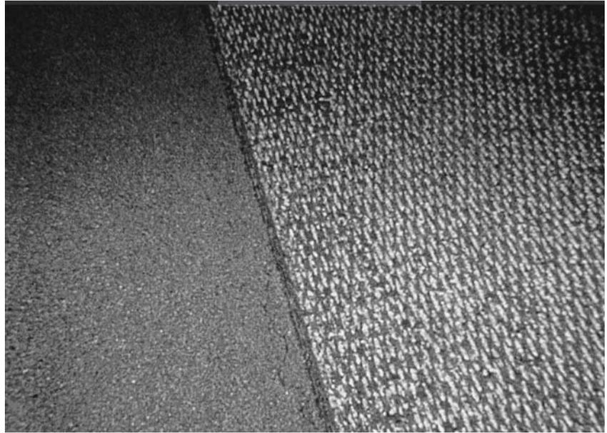
Milled Pavement Surface Improves Friction
