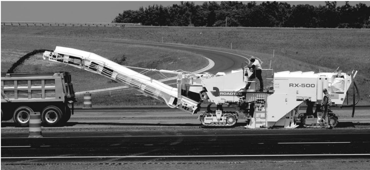
Typical Front Loading Milling Machine
